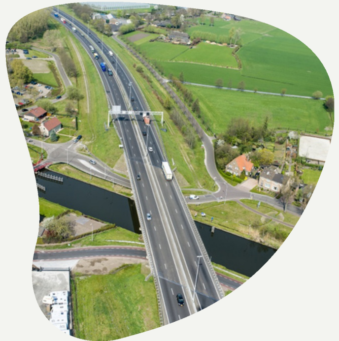
Wilhelminakanaal and highway A58, location of Oirschot
